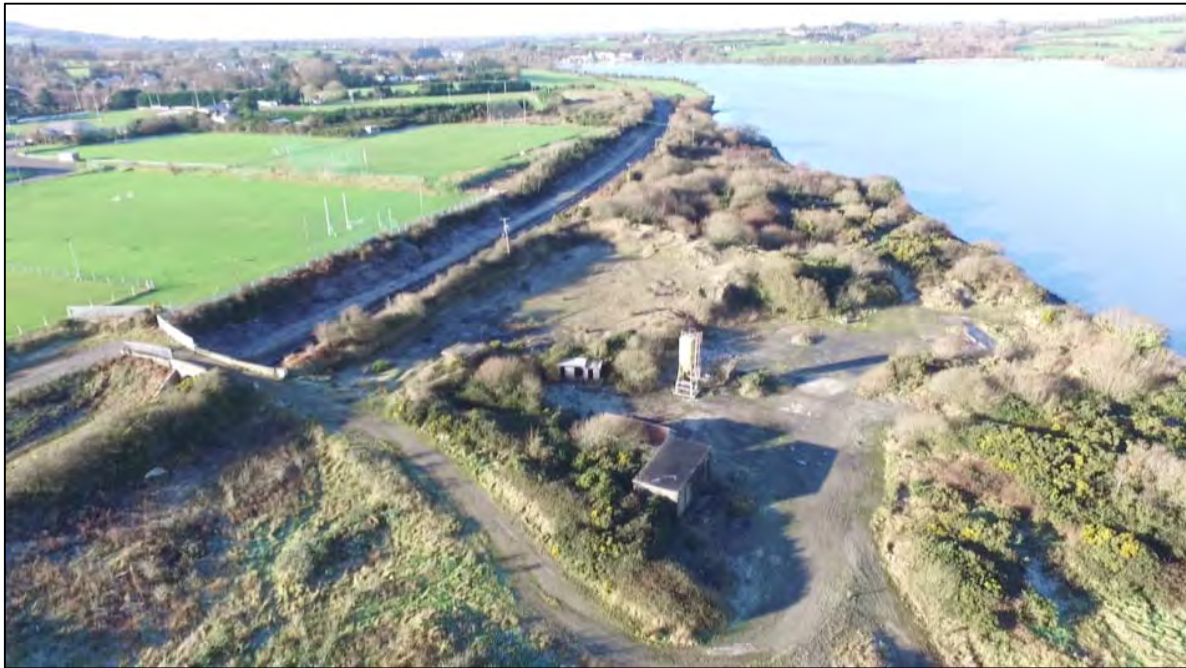
Photo 7.2.11 –View looking at western corner of site including abandoned quarry buildings
