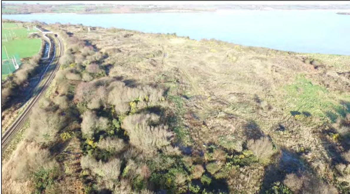
Photo 7.2.7 –View looking north-west
