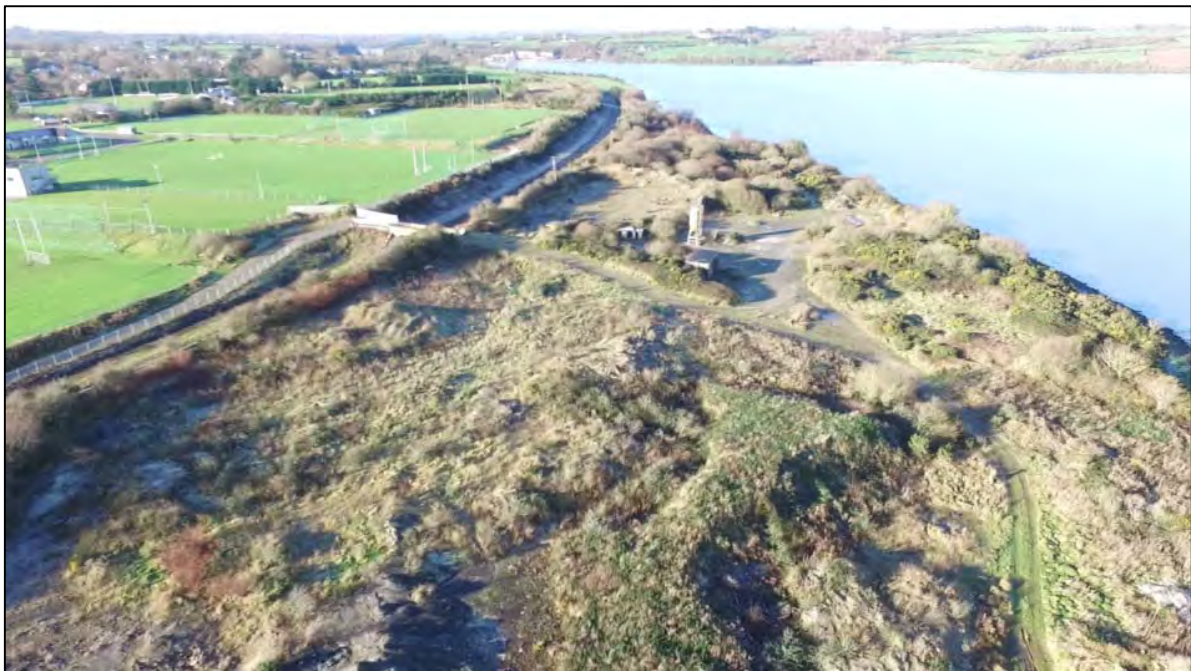
Photo 7.2.10 –View looking at western corner of site
